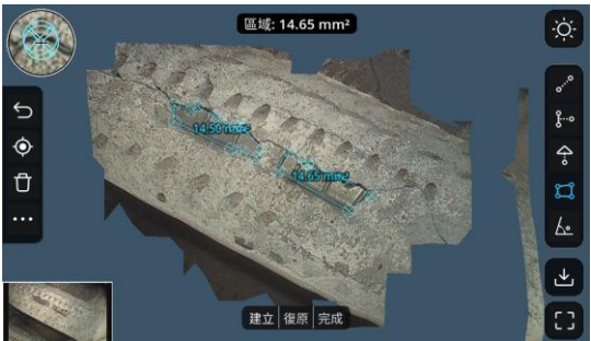
X3000 - 3D View Turbine blade inspection - 3D reconstruction
